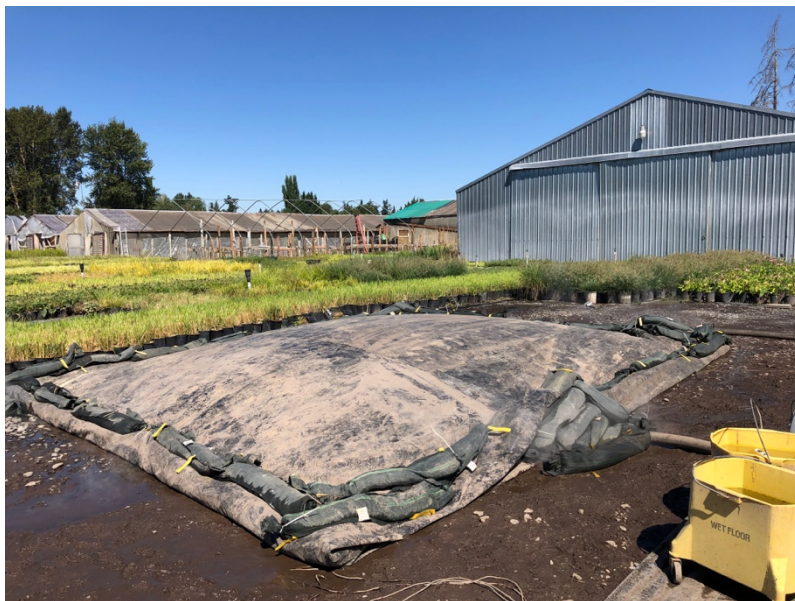
Figure 5. Steaming at a nursery with confirmed positive soil. This site had confirmed P. ramorum positive Arctostaphylos uva-ursi container stock that had been destroyed. Positive soil was also detected, and steaming was performed by ODA in August 2020.
