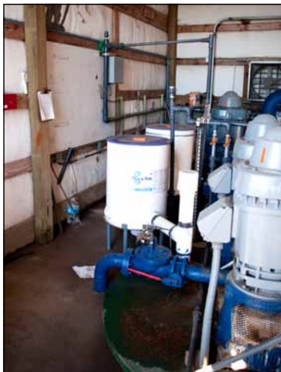
This nursery has a dedicated shed with chlorination treatment for disinfesting its irrigation water.
